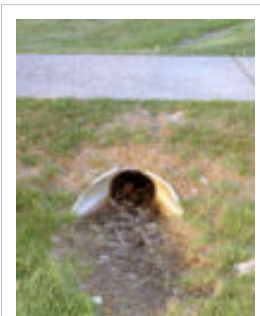
A small culvert under a pedestrian walkway.
